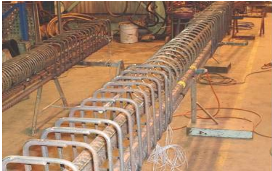
Figure 5.4(a) Fixing the helical reinforcement
