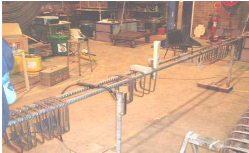
Figure 5.3(a) Measuring the spacing for stirrups and longitudinal reinforcement
