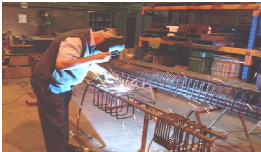
Figure 5.3(b) Fixing the stirrups and longitudinal reinforcement
