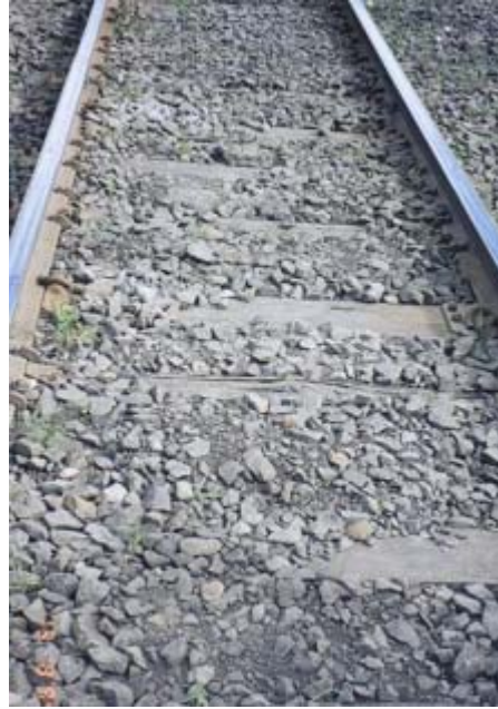
Figure 2.7 Track suffering from ballast degradation
