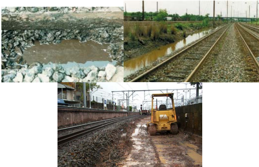
Figure 2.6 Tracks suffering from inadequate drainage
