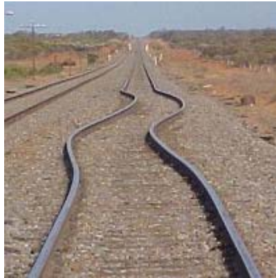
Figure 2.5 Inadequate lateral confinement can contribute to track buckling
