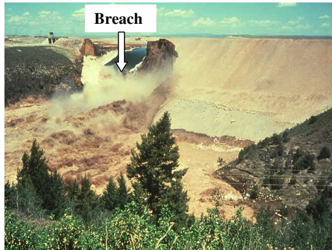
Figure 2.3 Failure of Teton dam due to piping in Idaho, USA
