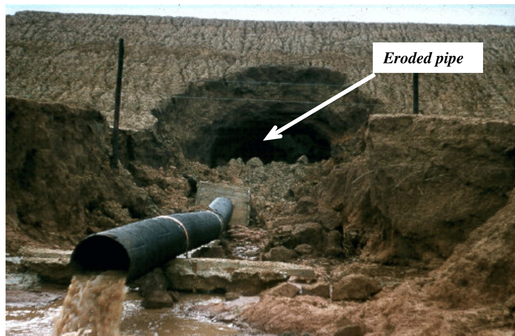
Figure 2.2 Piping incident of an embankment dam constructed with dispersive clay in Mississippi, USA ( www.fema.gov/library )
