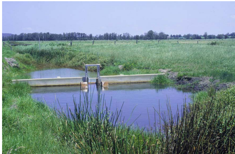
Plate 2.3 Self-regulating titling weir installed at drain P6D8, located on the western side of Broughton Creek.
