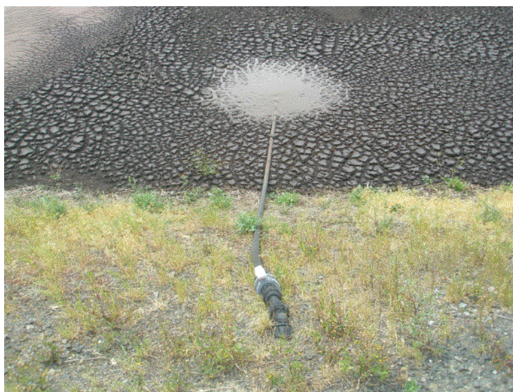
Figure 7.8 Residuals pumped out into the sand drying bed
