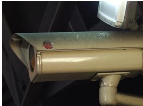
**Figure 7: Typical Dust Accumulation on VBFD CCTV Camera**
