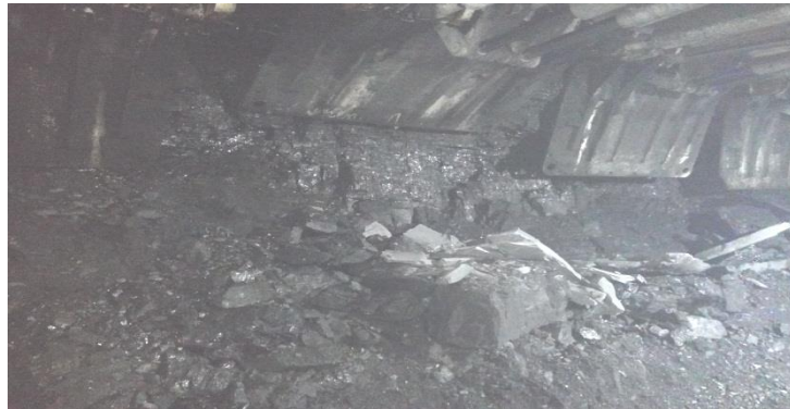
Figure 3: Rib spalling of LW12301 during first weighting
