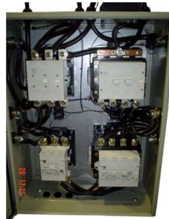
Figure 6. Test System Contactor Enclosure
