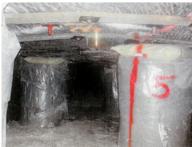
Figure 4 - Installation of pumpable cribs (Peng, 2007)
