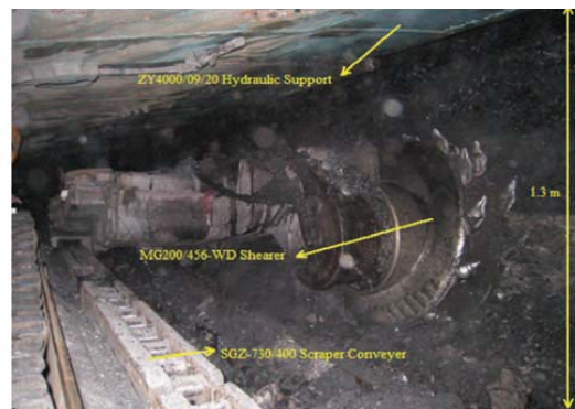
Figure 7—The longwall equipment in Qinan Coal Mine
