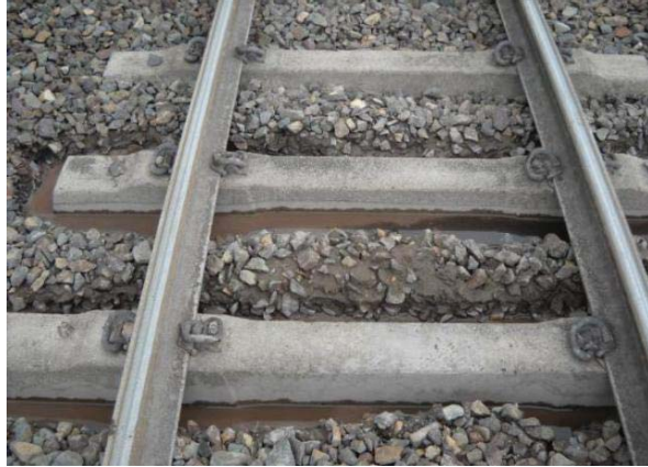
Figure 3: Mudholes caused by excessive coal/clay fouling (Goonyella System, QR National: Photo courtesy of Michael Martin)
