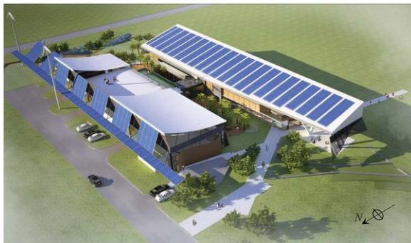
Figure 2 SBRC Building concept design showing wind turbines and PV arrays to north of high bay.
