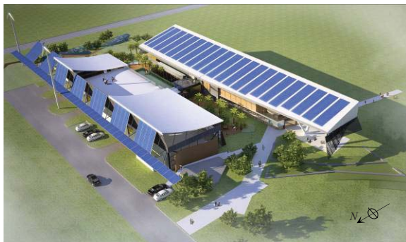
Figure 2 SBRC Building concept design showing wind turbines and PV arrays to north of high bay.
