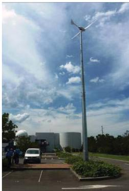
Figure 8 Aerogenesis 5kW wind turbine. One of two to be used to power the SBRC building, mounted on 18m articulated towers.
