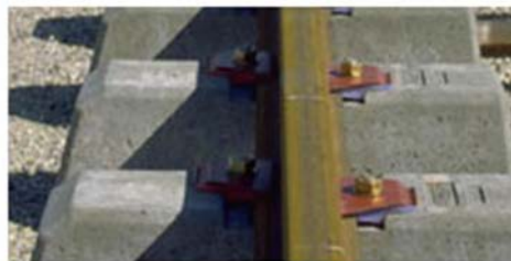
Twin Block Concrete Sleepers
