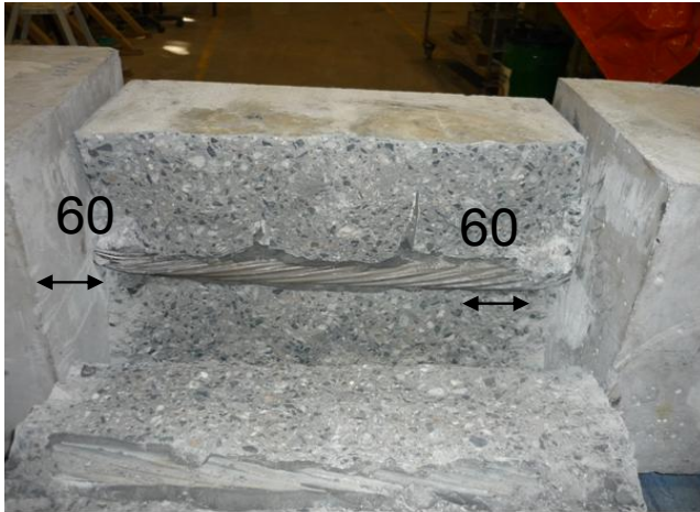
Figure 5. Concrete / grout crushing and cable bolt deformation in the vicinity.
