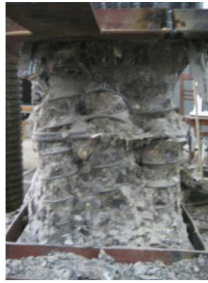
(b) Spalling of cover concrete
