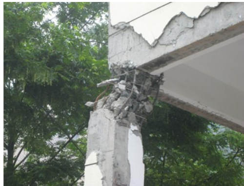
(c) Corner column
