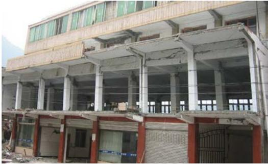
Figure 1. Failure at column ends
