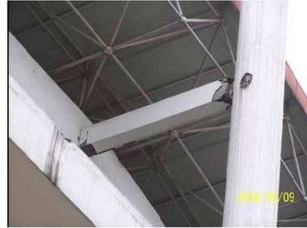
Figure 2. Failure at beam ends
