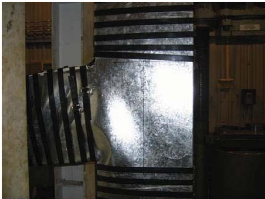
Figure 13 Buckling of galvanised steel
