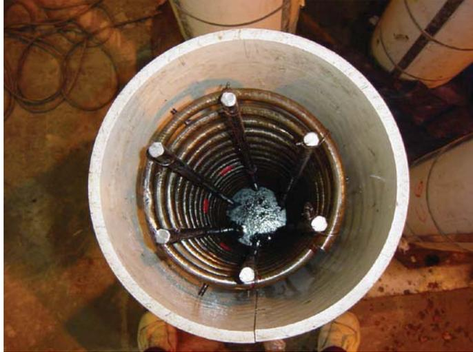
**Figure 2 – Placement of Reinforcement into formwork.**
