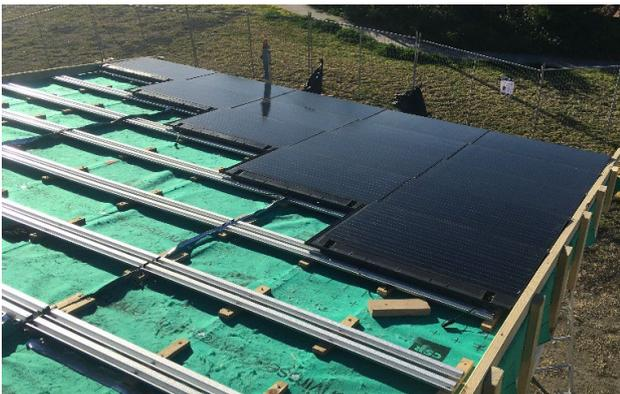
Fig. 4. Desert Rose house BIPV solar roof
