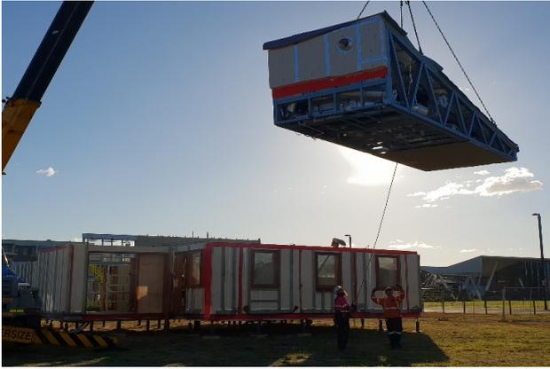
Fig. 3. HVAC cage installation
