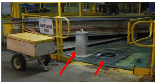
Image 2: As 2 O 3 trolley, chute and sample opening (Roseberg 2014)
