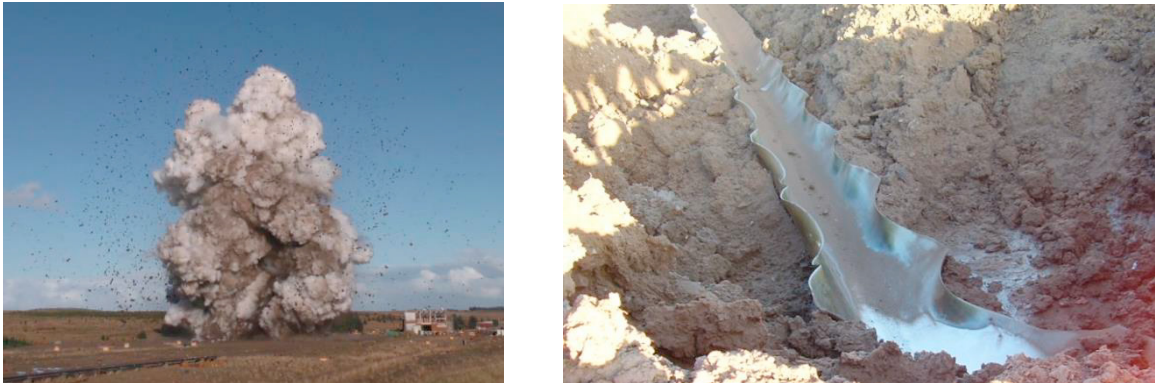
Fig. 3. A view of the explosion from the ENE direction, and the fractured pipe and crater formed by the pipeline rupture
