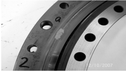
Picture 7 (a) A view of damaged rollers in axial plane (b) Outer raceway damage
