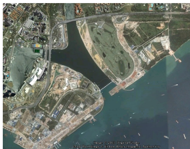
Figure 4. Location of the marina barrage.
