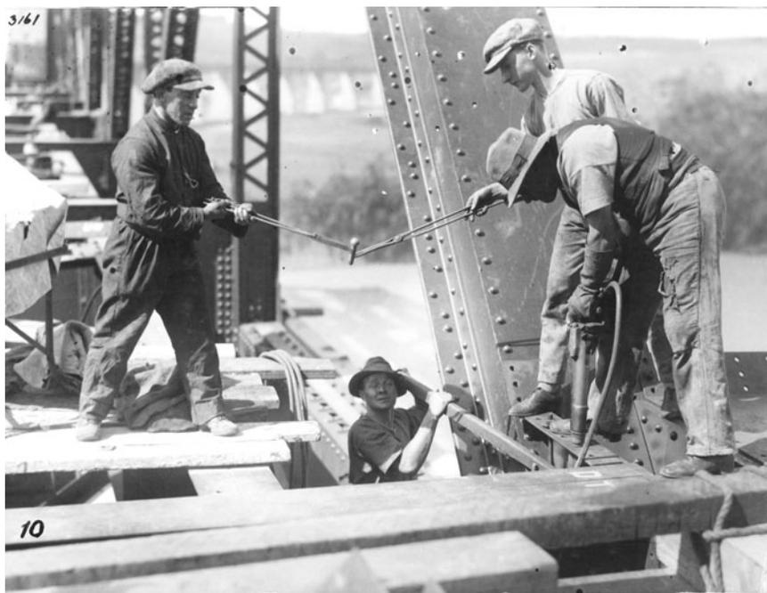
Figure 1. Riveters building the Murray Bridge, New South Wales, early twentieth century. State Library of South Australia; image no SLSA: B 3 161. Used with permission.
