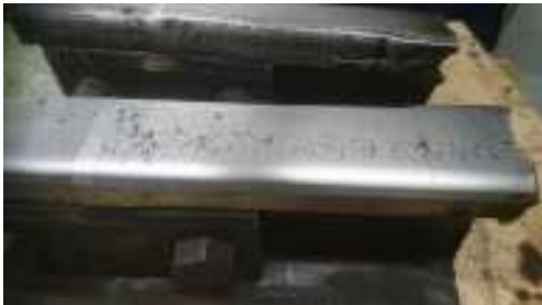
Photo 1 – Rail head cleaned and ready for inspection.
