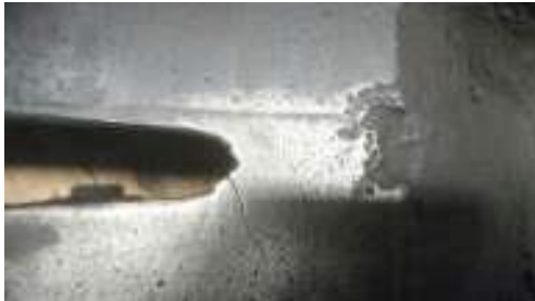
Photo 4 – Fracture site as viewed from below.
