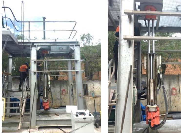
Figure 1: DSI Underground drill rig (grouted cylinder positioned above rig – left image)
