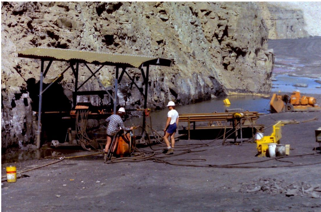
Figure 3: In-seam drilling in German Creek open-cut mine (Hungerford, 1988)
