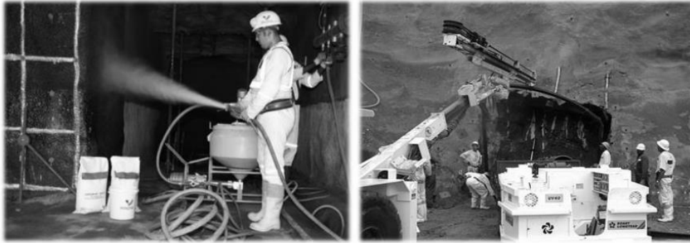
Figure 4: Photos of TSL application and shotcrete (Jjuuko and Kalumba, 2014)
