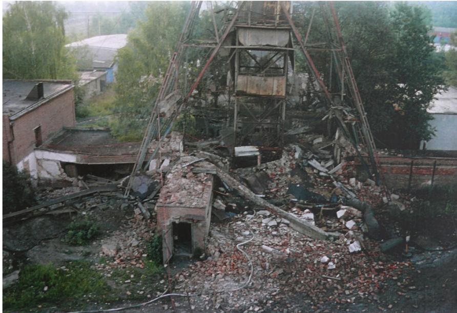
**Figure 1: Gas explosion at Hermanice Mine during the liquidation of the He-III shaft**
