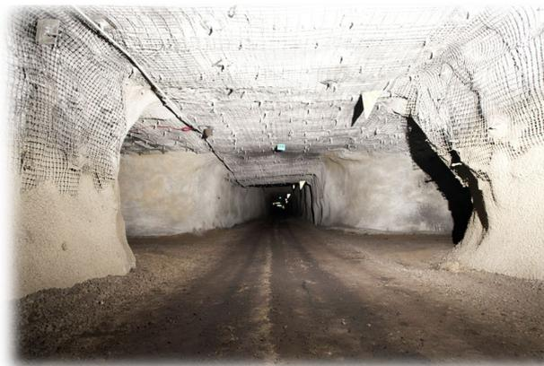
**Figure 2: Underground Intersection rib support with FRS**
