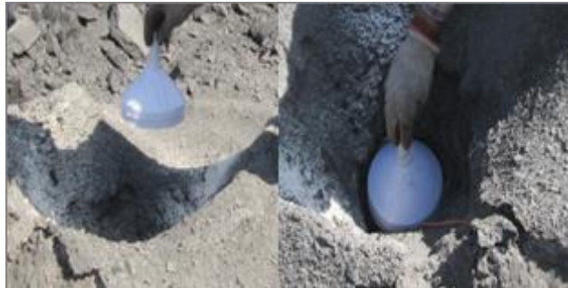
Figure 4: Inserting reverse plastic funnel in blast hole
