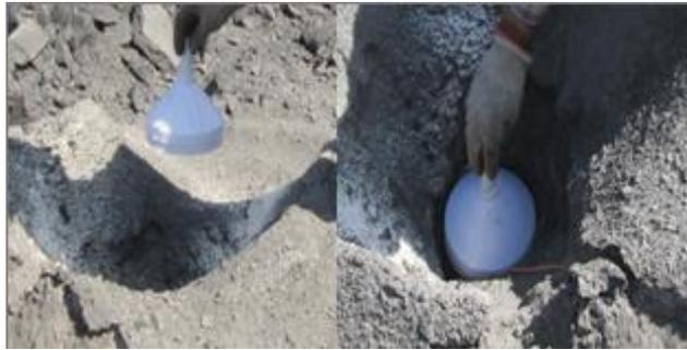
**Figure 4: Inserting reverse plastic funnel in blast hole**
