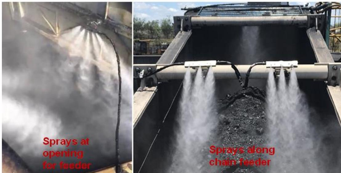
**Figure 6: Installed dust suppression system at exit of hopper, along chain feeder and at transfer from chain feeder to primary sizer**
