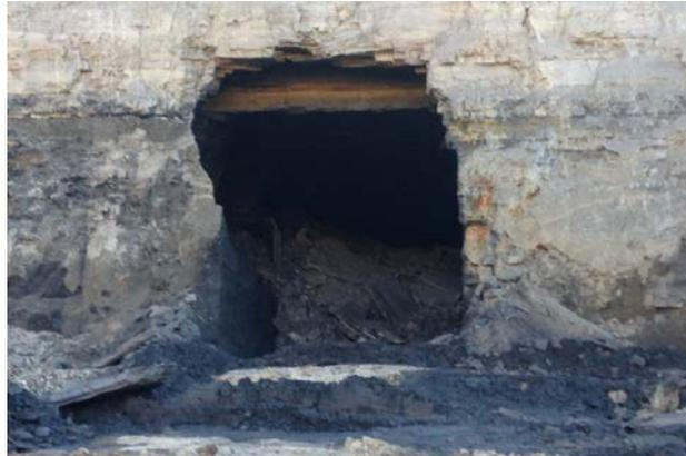
**Figure 8: Time based decay of entry due to ingress of water**
