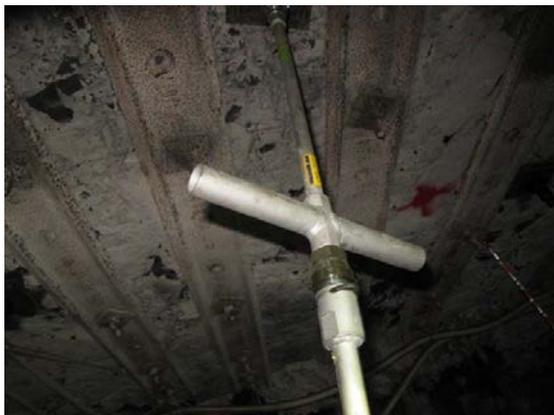
Figure 20: Grout lance attachment
