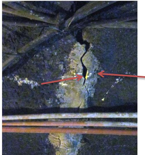
**Figure 4: Squeezing of surrounding rock mass after installation of steel ribs.**
