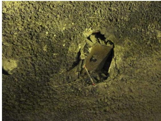
**Figure 3: Squeezing of surrounding rock mass before installation of steel ribs.**
