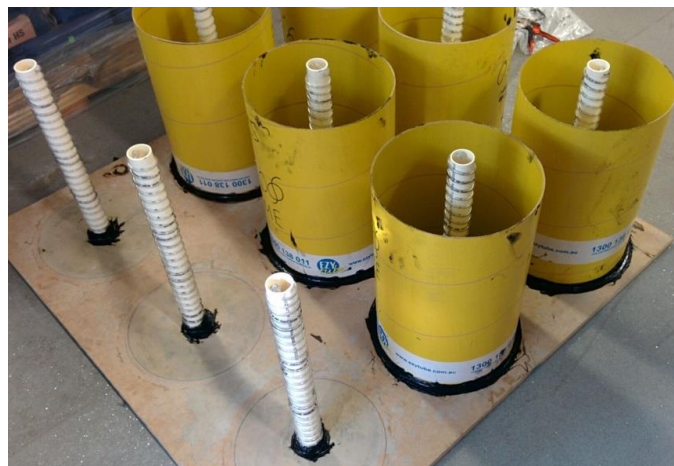
Figure 4: Completed moulds ready for casting
