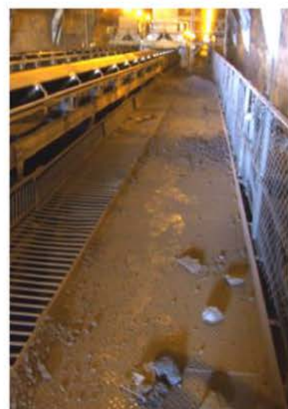
Figure 6: Coal Bunker Walkway
