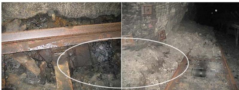
Figure 9: Damage to dolly-car rail & spalling in the conveyor drift
