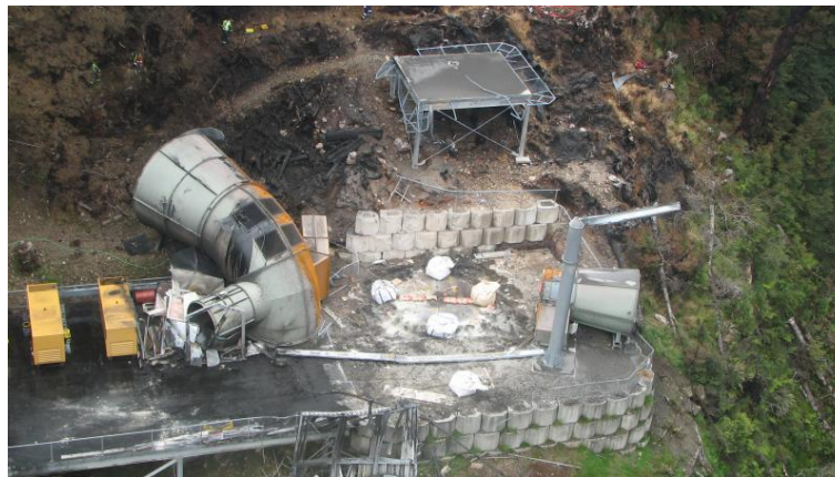
Figure 4 - The capped fan shaft, showing the evasee where it was deposited after the fourth explosion (NZ Police, 2012)
