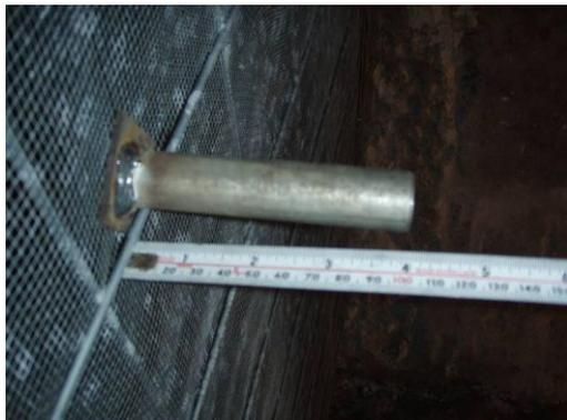
**Figure 3 - Depth indicator attached to Tecmesh sheet formwork**
