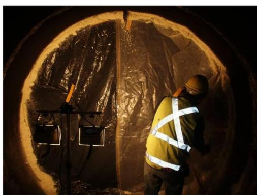
**Figure 6 - Plastic curtain to seal gas volume**
