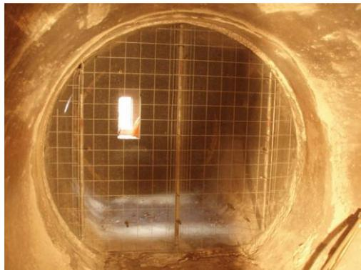
**Figure 4 - Formwork for 100 mm seal**
