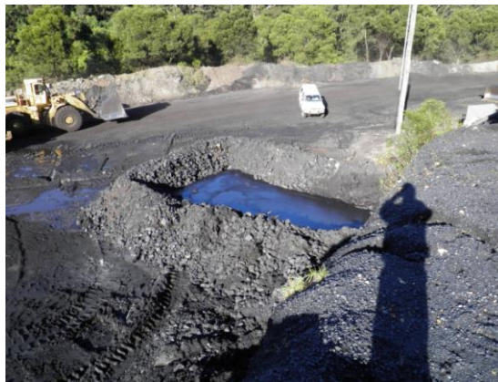
Figure 6 - Dam composed of loose rocks
