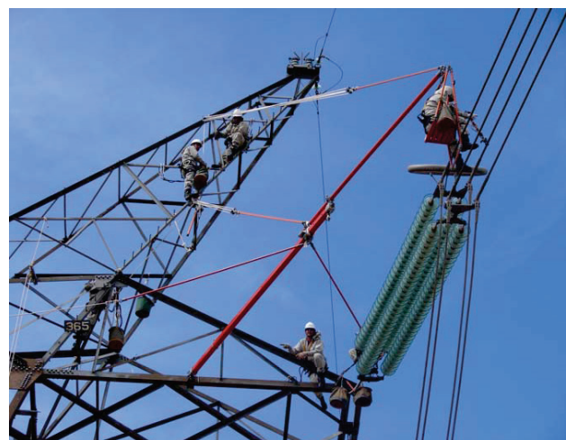
Figure 1 Changing 765 kV insulator string using Bare Hand Method in Brazil [5]
