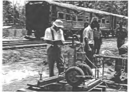
Fig. 6 Using A Cone Penetrometer Test to Re-Classify the Soil Profile at the Site of the Catastrophic Train Derailment
