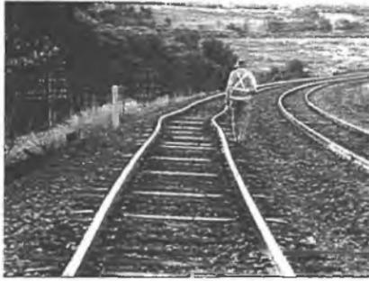
Fig. 28 Track Buckling due to Stress Build up in the Welded Rail as a Result of Heat and Insufficient Lateral Stability to Hold the Track
