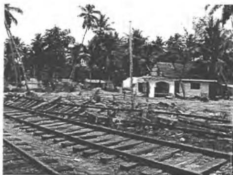
Fig. 9 Passenger Rail Track Reconstructed after Tsunamis Occurrence without Appropriate Subgrade Improvement (near the City of Galle, Sri Lanka)
