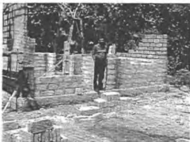
Fig. 15 Constructions of Walls with Concrete Bricks, during Reconstruction
