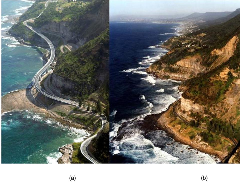
Figure 3. The Sea Cliff Bridge constructed as risk management solution to ongoing rockfalls, debris flows and landslides. b The original slopes with problematic Lawrence Hargrave Drive near base of cliffs between Coalcliff and Clifton.
