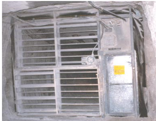
FIG. 22 - An example of a louvre regulator.
