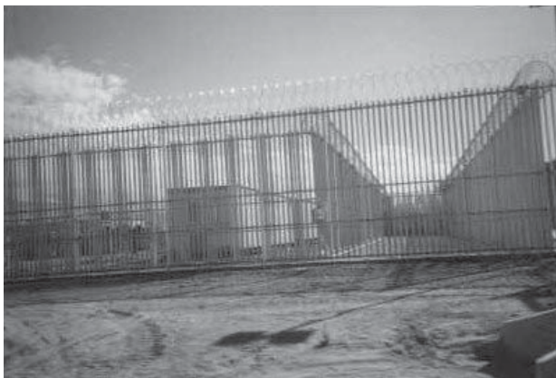
The Oscar compound, Woomera, South Australia, January 2002
