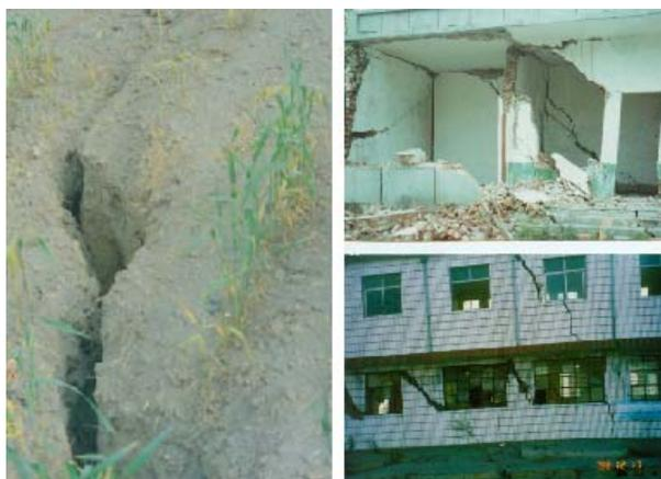
Figure 2 - Farmland and structures damaged by mining
