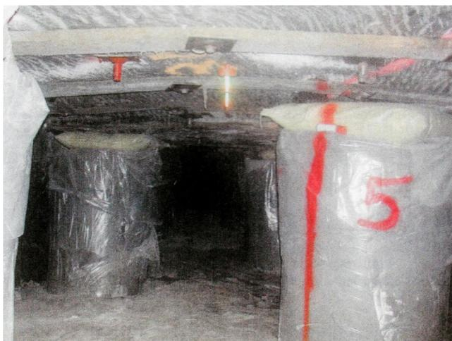
Figure 4 - Installation of pumpable cribs (Peng, 2007)
