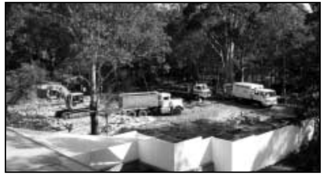
Construction begins on the new UniBar
