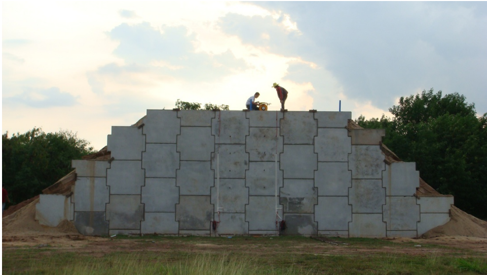
Figure 4: Full-scale test BRE wall.
